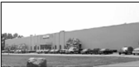
BIW Cable (Draka) cleaning services provided at offices and plant.
